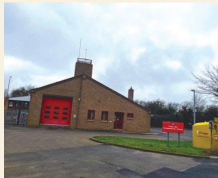
Corby Glen Fire Station
