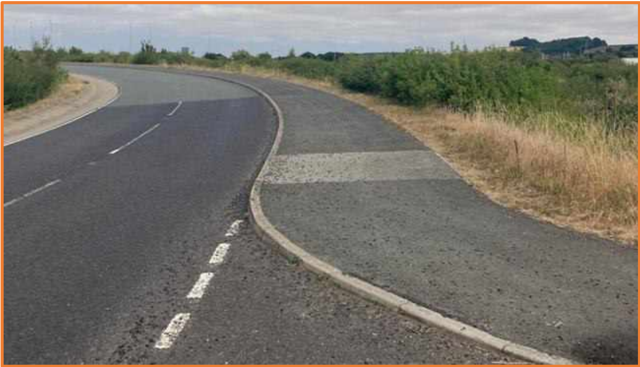
Figure 4: existing shared footway/cycleway on the southern side of Gonerby Lane, looking north towards the A1
