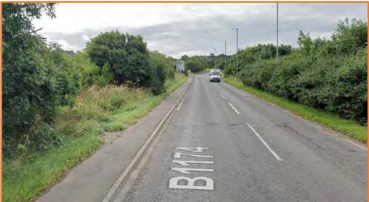
Figure 5: existing footway along the B1174, looking south towards Great Gonerby
