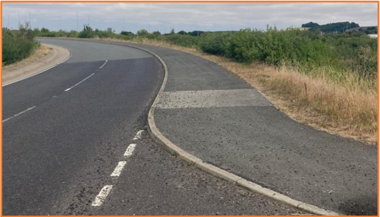
Figure 4: existing shared footway/cycleway on the southern side of Gonerby Lane, looking north towards the A1
