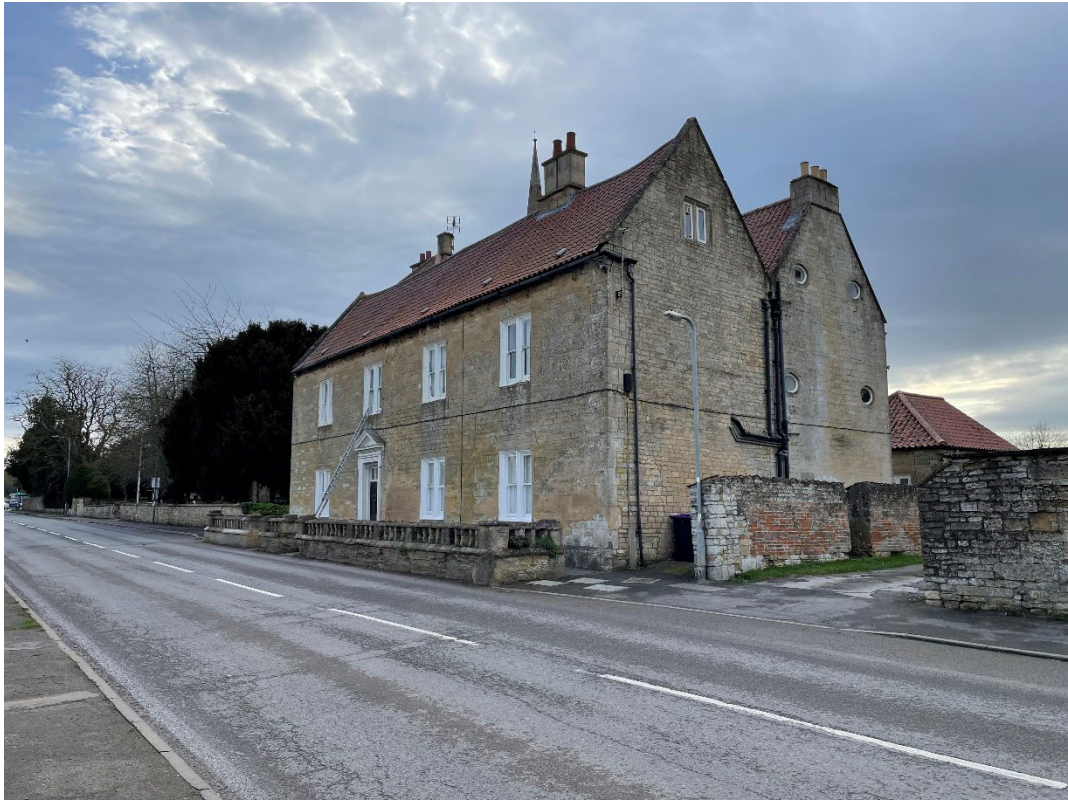
Plate 8 Ancaster Hall, looking south-west
