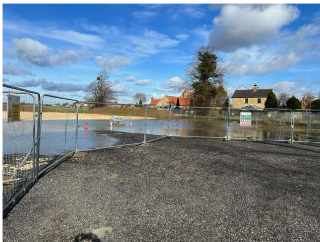
Two photos taken 23/2/2024 of the pipeline flooding adjacent to Dickens Close
