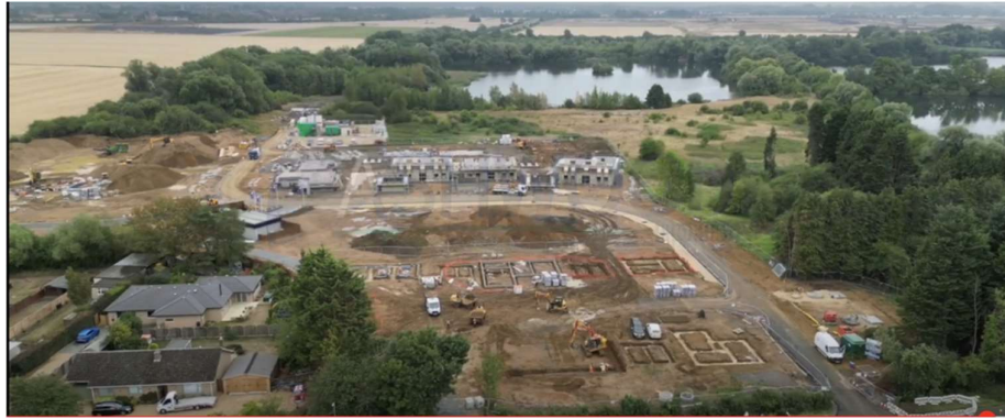
Figure 6 Teal Way Example of scale of works
