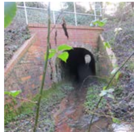
Figure 11: Existing brook and culvert beneath the railway line
